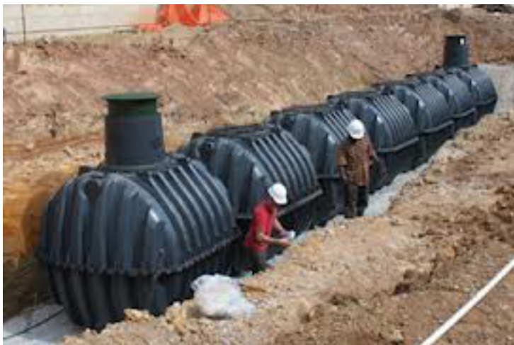
A similar system to the one in the photo was installed at MassMutual.
